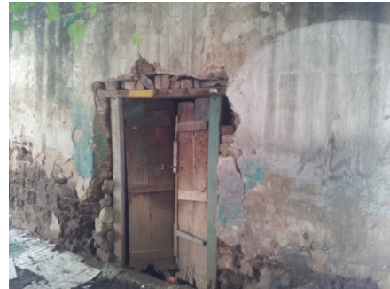
Figure 21. Exterior View– Hindu temple In Kashmiri Bazar
