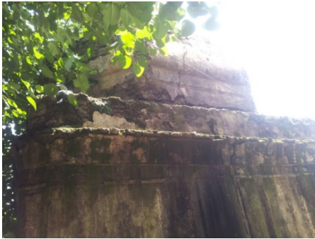
Figure 20. Exterior View– Hindu temple In Kashmiri Bazar
