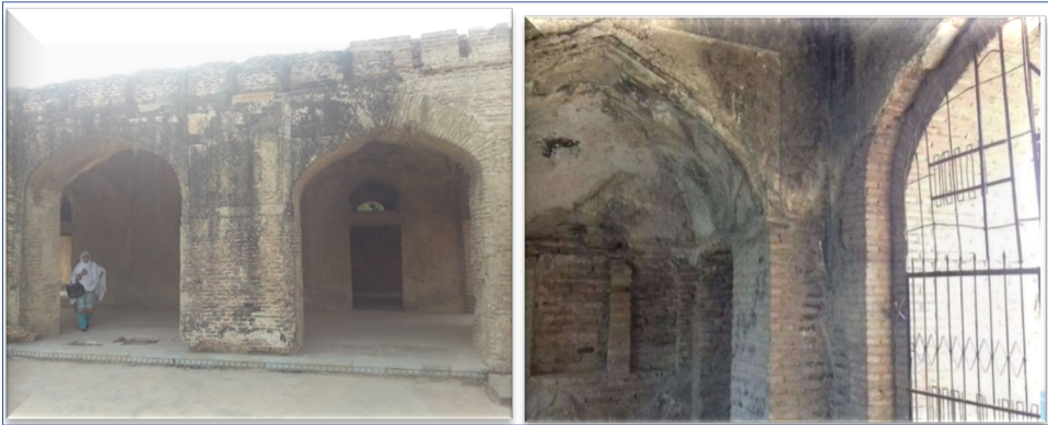
Figure 7: Baradari - Four Centered Arches
