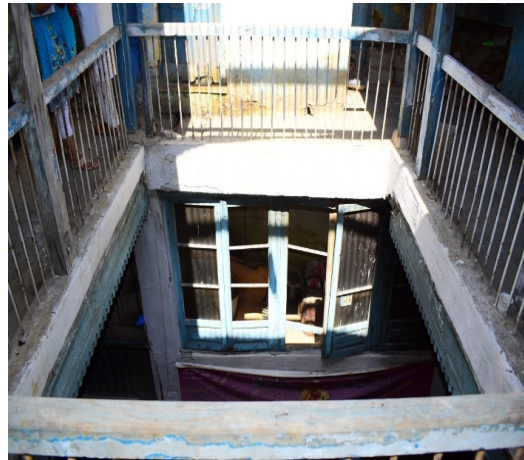
Figure 20: View of the gallery with direct sunlight
