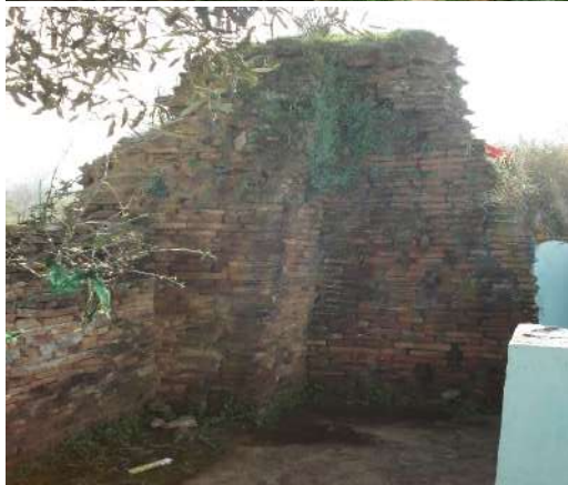
Figure 1: A View of Hallowed and Solid Bastions at Naukot
