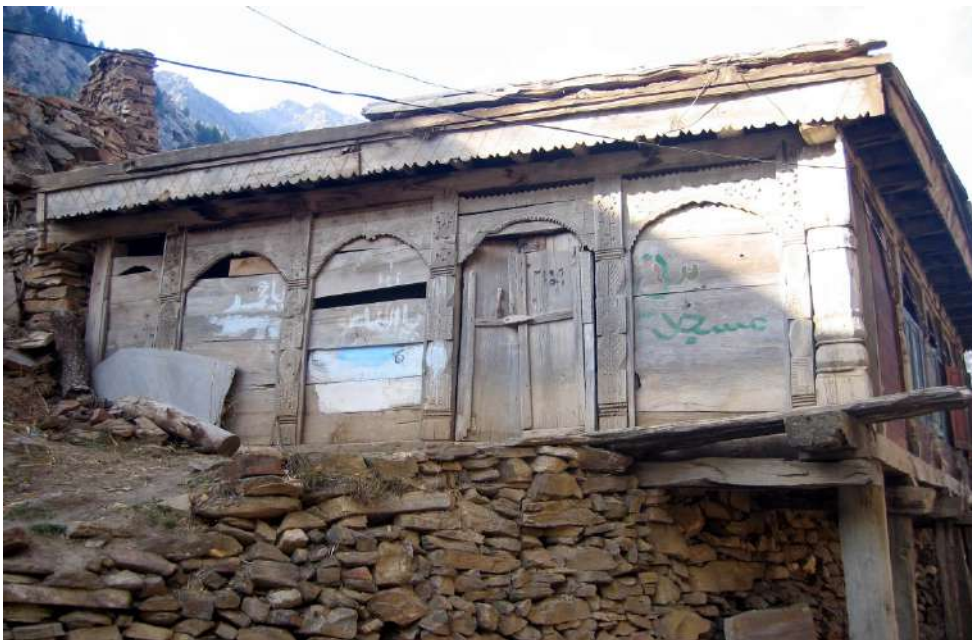
Figure 3: General View of Bela Mosque Overlooking northeast
