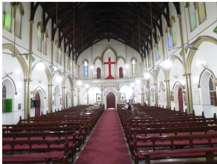
View of Gallery, Nave, Colonnade, Clerestory, Scissor Roof, and Seating in St. Mary Magdalene Church Lahore Cantt.
