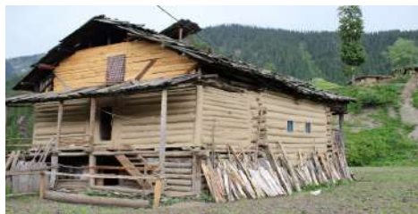
Figure 19: Wood log and Plank Construction
