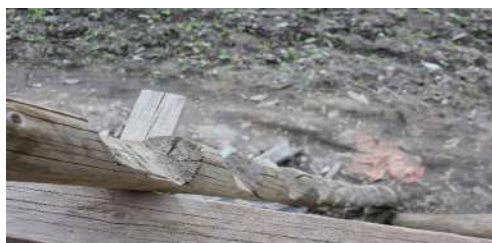
Figure 20: Ladder to Access the Rear Terrace
