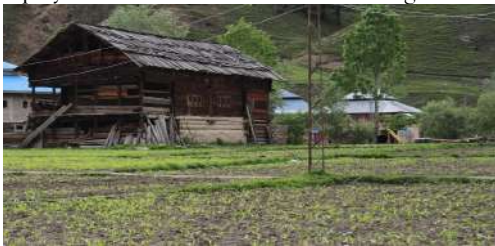
Figure 22: Wooden Planks as Roofing Material
