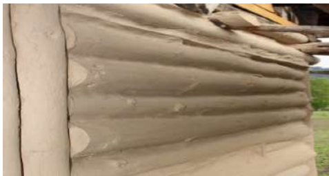
Figure 23: Wood log Walls and Mud Plaster
