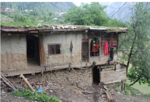
Figure 5: Front view of the House
