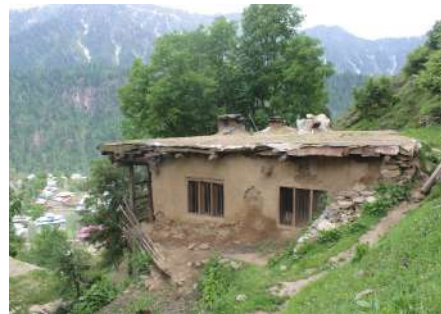
Figure 14: Flat Roofed House
