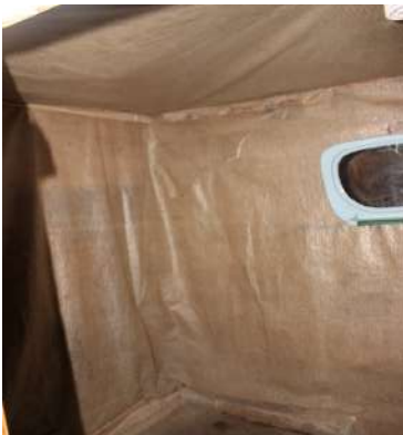
Figure 28: Water Proofing in Bathrooms
