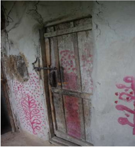
Figure 8: Doorway and Plaster Details
