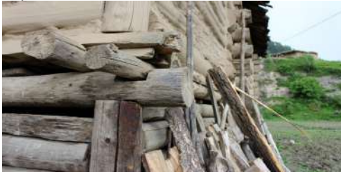
Figure 21: Interlocking Wood logs as Structural Elements
