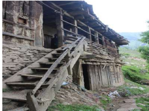
Figure 6: Access to the Upper Floor
