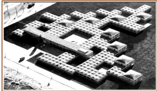
Figure 2: The Municipal Children's Home, Amsterdam 1960 by Architect Aldo van Eyck. Source: (Strauven, 1998).
