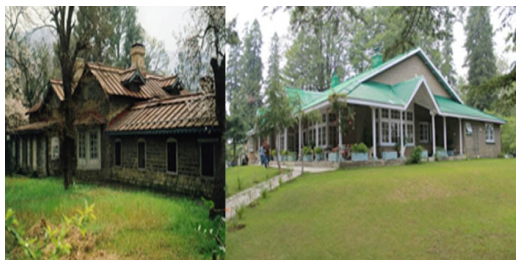
Figure 5: Colonial houses in Abbottabad
