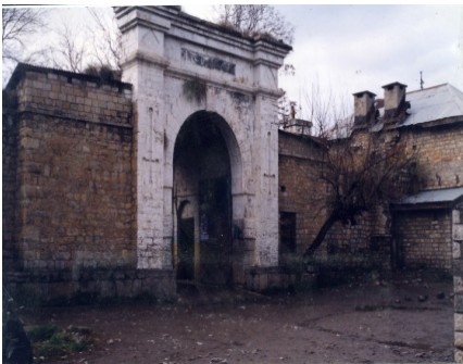
Old Tehsil Building
