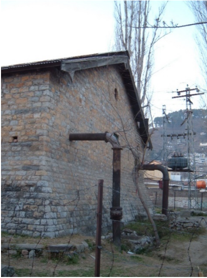
Stone Built Water Tanks
