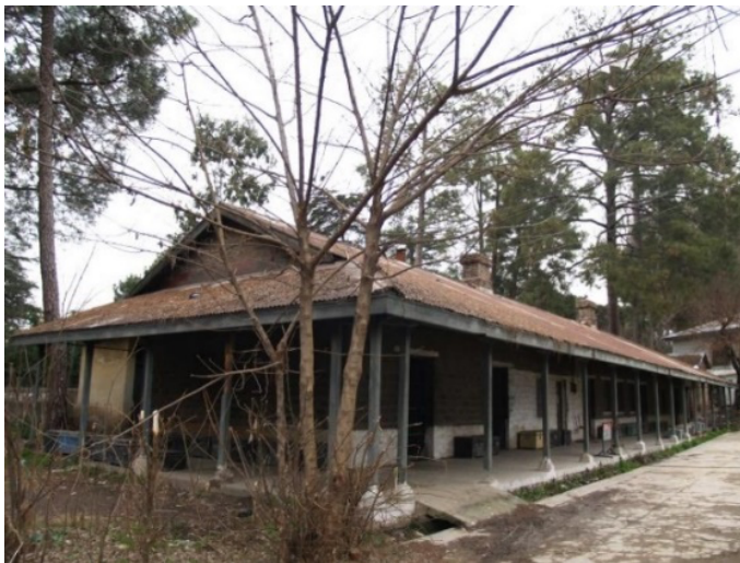
Strong Room Hut
