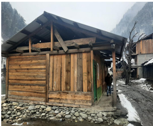
Figure 6: Existing Wooden Structures in Tehjian Market
